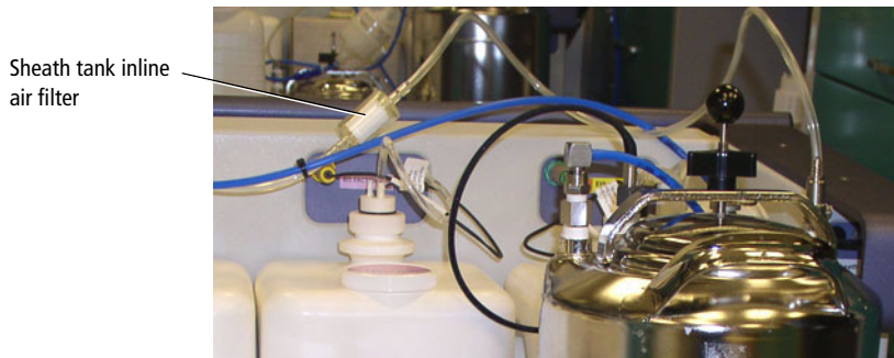
Figure 6-19 Inline air filter for sheath tank
